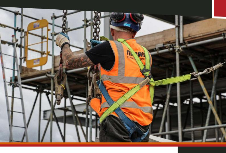
Fall arrest is the last method of work at height control measure that should be considered because everything should be done to avoid falls altogether. But sometimes it is the only possible solution. All of our lift teams come equipped with this system at no extra charge and we attach it to our crane hooks which has the added advantage of an integral method of rescue.
