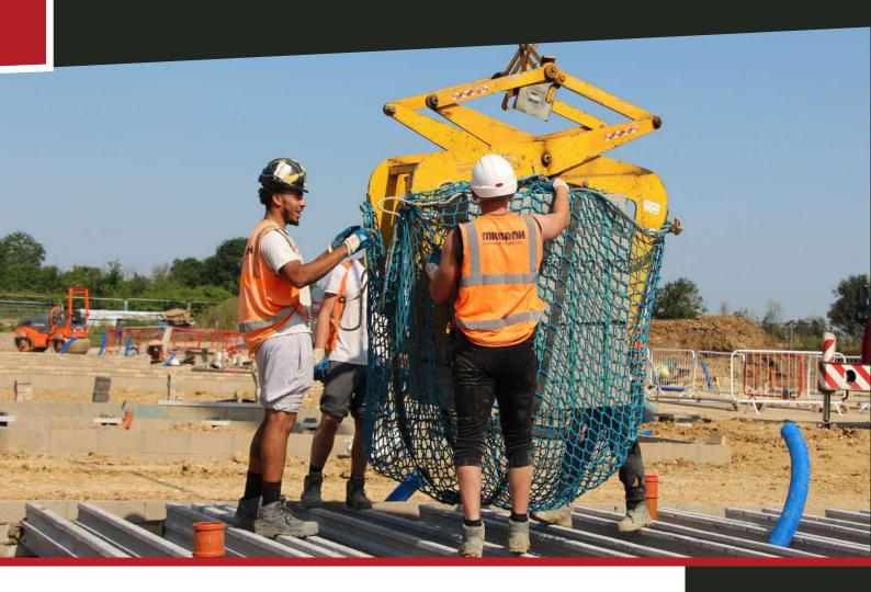
In traditional house building concrete blocks are one of the most common materials and they are delivered in packs of 48 or 72. The block grab and safety net is the only safe way to lift these packs and avoid the risk of injury and disruption.
