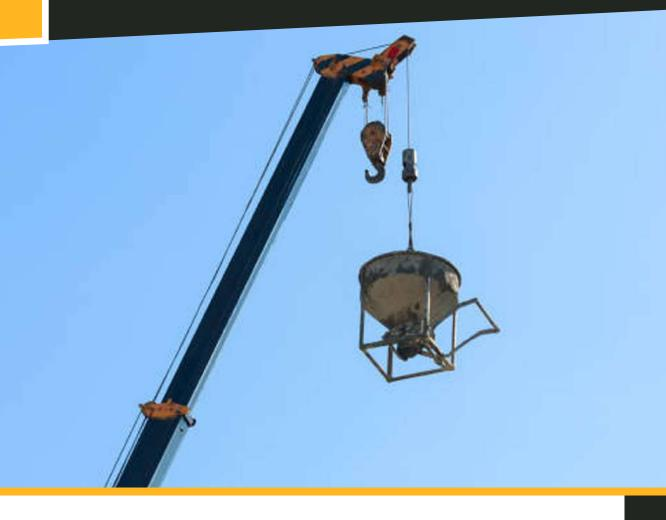
Reinforced concrete cast on site is still a very popular form of construction but it is not always possible to deliver concrete where its needed. Concrete pumps are one solution and the other is to lift it using a crane. When lifting using a crane you need a strong, versatile container that can be discharged safely and efficiently. The concrete skip is ideal and comes in various sizes and configurations.
