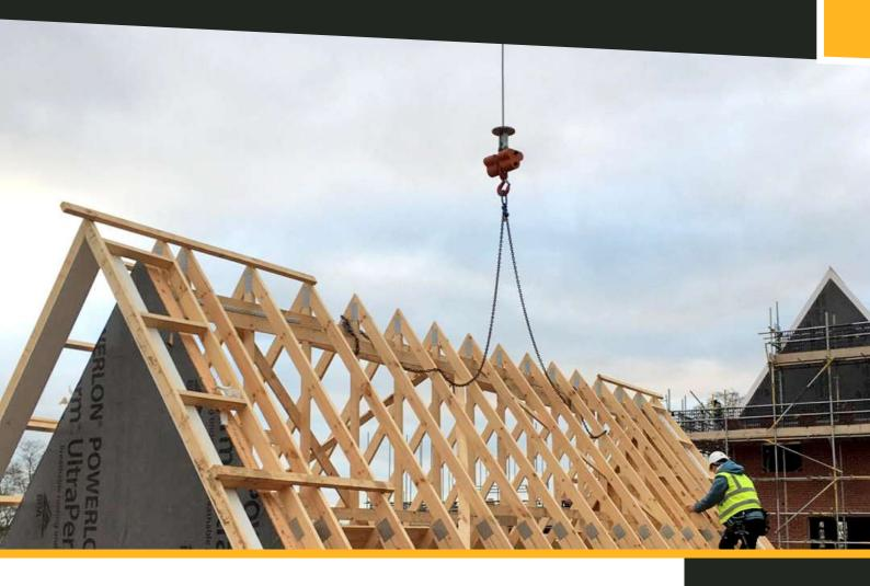
We are in one of the busiest regions in the country for housebuilding and where there are houses there are roof trusses. We lift tens of thousands of trusses every years and this simple attachment makes the process considerably safer, removing the need for awkward, unplanned work at height required to attach lifting chains and slings. They are so effective, we have one on every crane.
