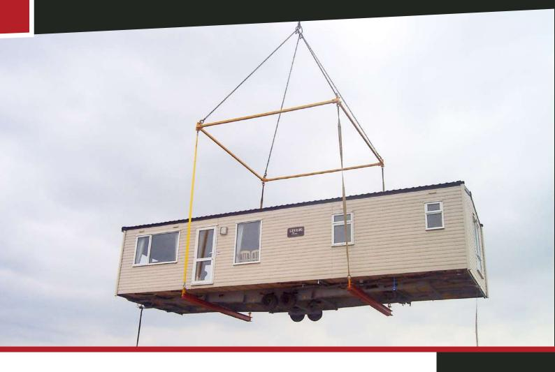
It is surprising how regularly we are asked to lift these 'mobile' homes. The problem is, they are not designed for to go up and very difficult to lift without causing substantial damage. For this reason many crane companies refuse to get involved. But that is not the Cadman way. Instead we developed, manufactured and tested a system of beams and spreaders that allow us to lift many types of caravan safely, quickly and without damage.
